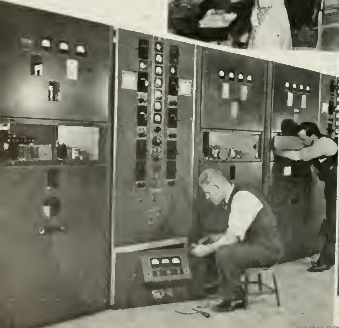
A 5-KW. HIGH FREQUENCY COMMUNICATION TRANSMITTER NEARS COMPLETION.
